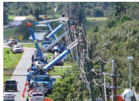
Top left and above left: Duke Energy crews work to replace two 40-foot poles and a pad-mounted transformer that Hurricane Milton destroyed in Florida. Top right: Tampa Electric rescue work before the storm surge had receded. Middle right: Members of Minneapolis Local 160 gathered before working in Georgia. Above right: DTE trucks at a refueling stop on the way to Georgia. Above middle: Local 1245 crews in Florida.
