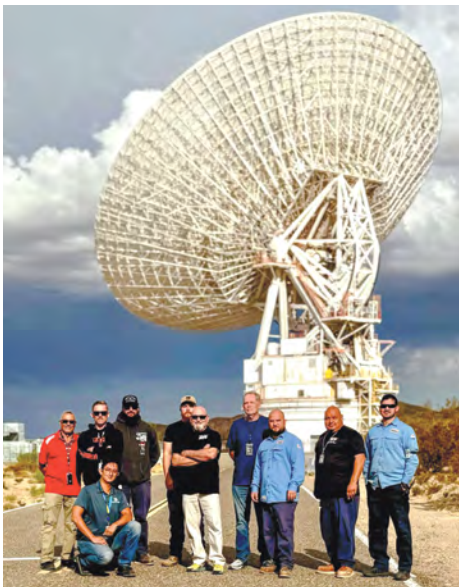
Local 543 members keep NASA's massive satellite dishes at Goldstone communicating with the agency's extra-terrestrial network of spacecraft and landers.
